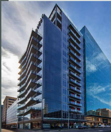
PwC Building Quest on Franklin
